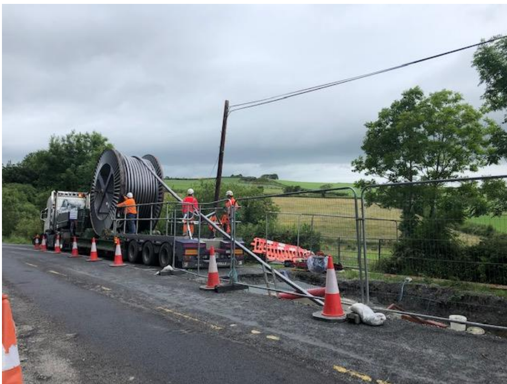
Figure 2-9: Typical cable pulling at a joint bay
