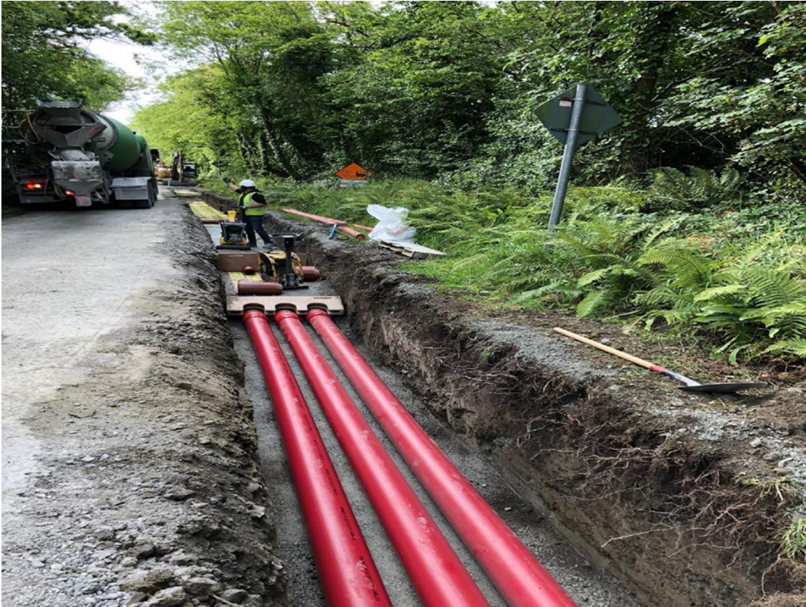
Figure 2-6: Typical Cable Trench in Road
