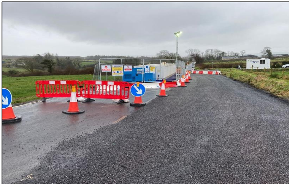
Figure 2-3: Typical passing bay around a joint bay
