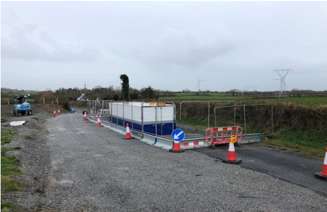
Figure 2-10: Typical HVDC Cable Jointing Bay Shelter
