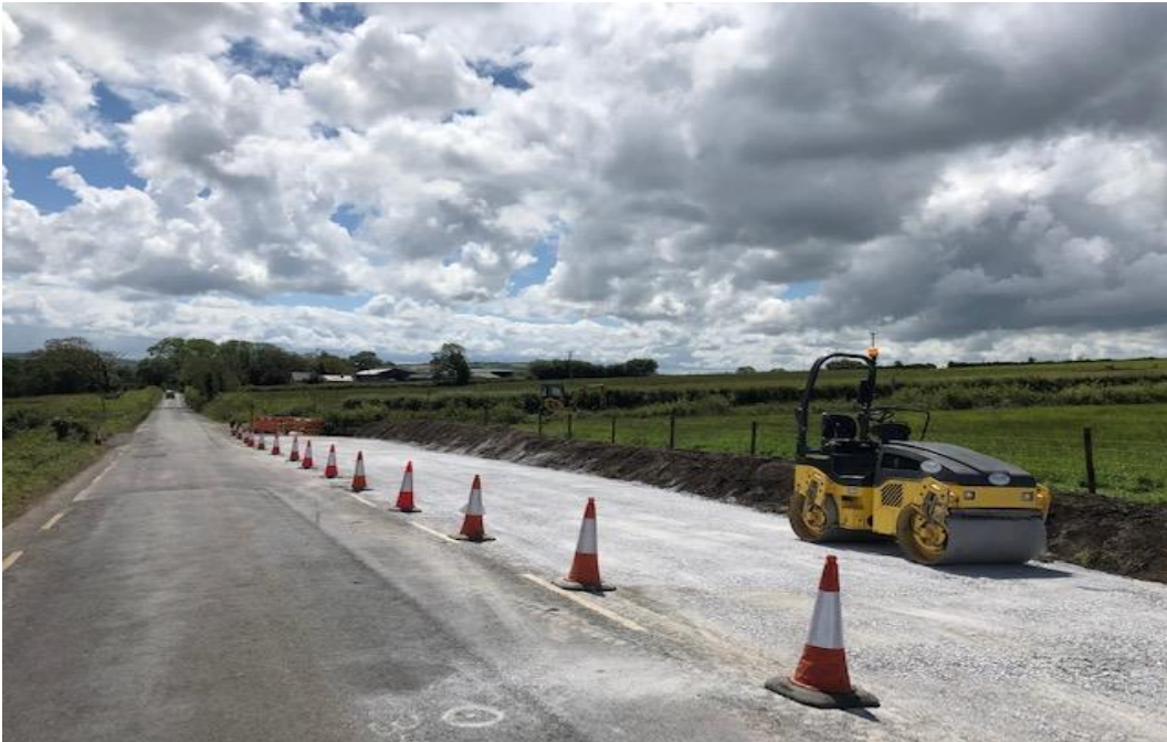
Figure 2.10: Passing Bay (on the Kilpaddoge Knockanure 220kV UGC Project, Co. Kerry – refer)
