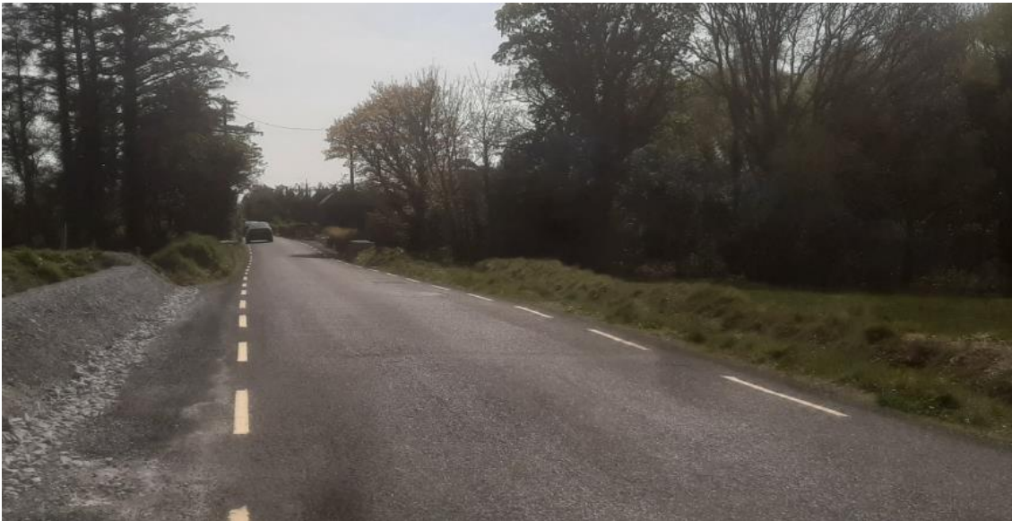
Figure 2-7: Reinstated road following laying of UGC
