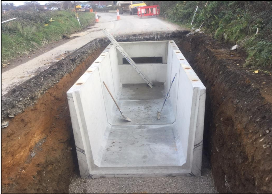
Figure 2-1: Typical joint bay
