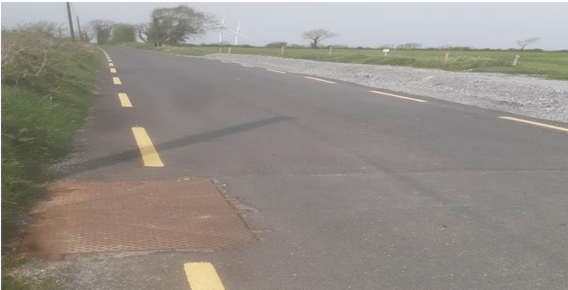
Figure 2-2: Reinstated road at joint bay (darker tarmac) with communications chamber
