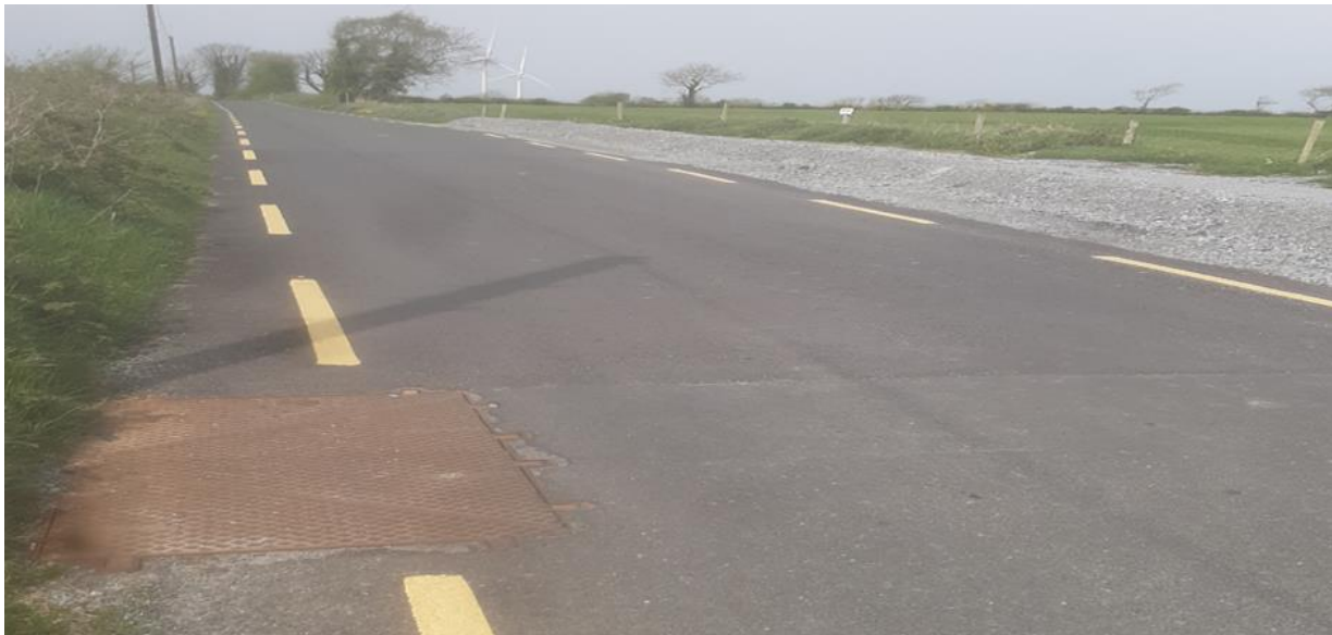
Figure 2.3 Reinstated road at joint bay (darker tarmac)
