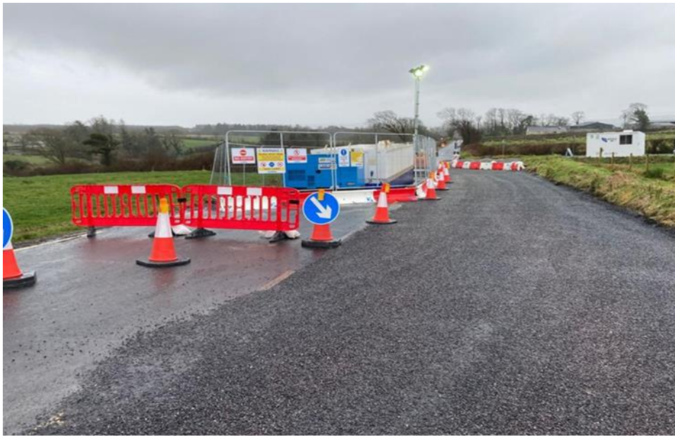
Figure 2.4 Typical passing bay around a joint bay
